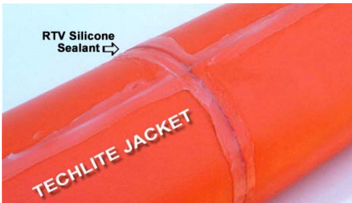
Photo 1: All seams over sealed with RTV
