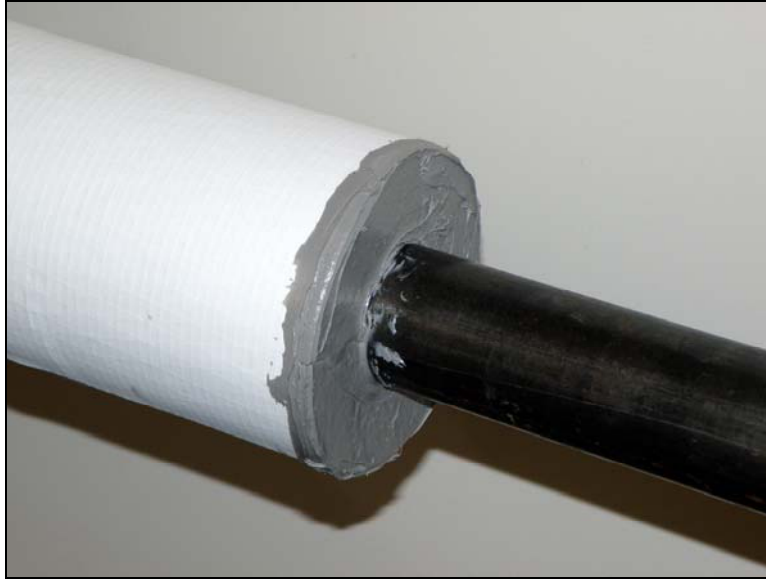
Photo 2: Butt joint vapor sealing
